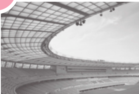
Tsutsunaka Plastic Industry's "SUNLOID PC" is widely used in domes, window canopies and other structures for natural lighting.
