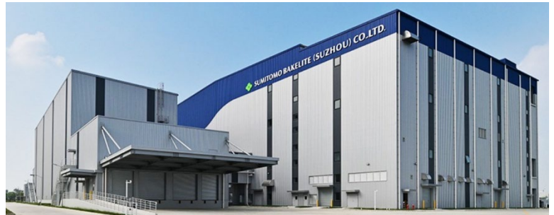
New Plant for Semiconductor Encapsulation Materials at Sumitomo Bakelite (Suzhou) Co., Ltd. (Completion: 2024)
