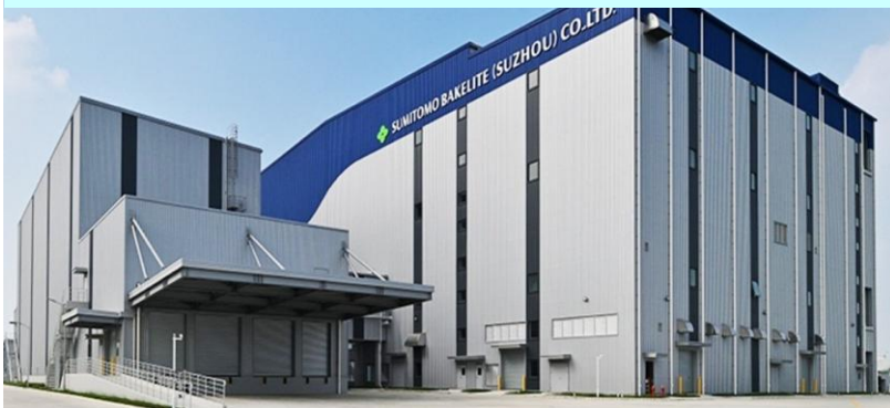
Suzhou New Encapsulants Materials Plant (completed in 2024)
