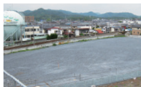
Site following the completion of the remediation work (May 2009)
