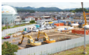
Overall view of the remediation work (June 2008)
