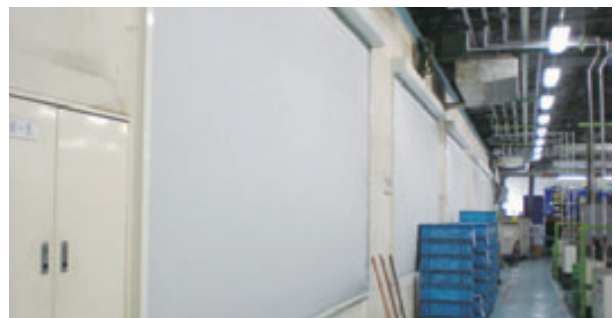
Light shield installation (Tsu Plant)
