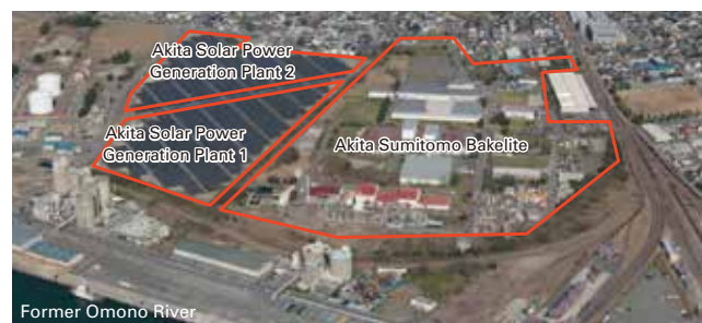
Aerial photograph of the facility
