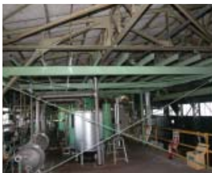
Structural reinforcement as an earthquake countermeasure (Shizuoka Plant)
