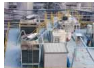
Water recirculation equipment (Amagasaki Plant)
