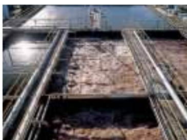
Activated sludge process equipment (Shizuoka Plant)
